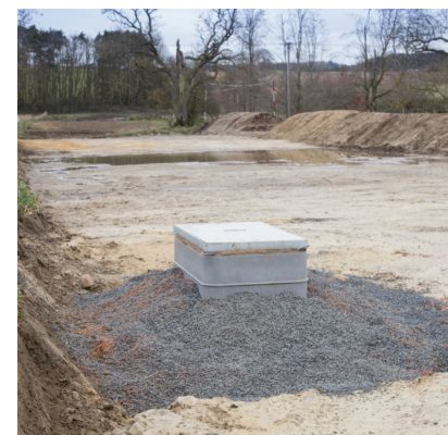
Cable easement prior to reinstatement, with link box
