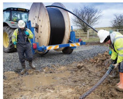
7. Pull cables into ducts
