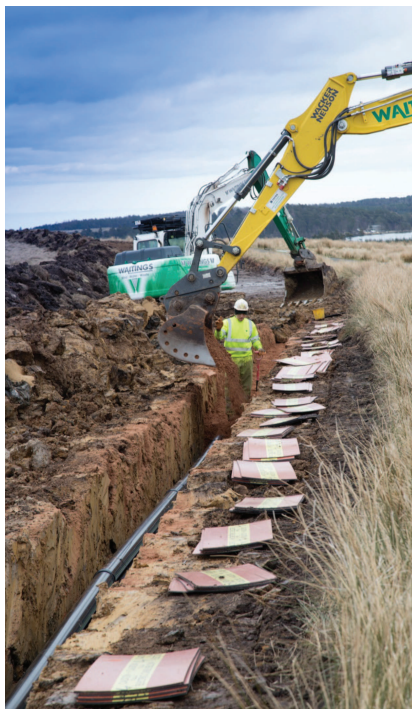
3. Ducts Covered and Protective Marker Tiles Laid
