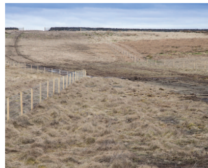
5. Reinstatate Topsoil
